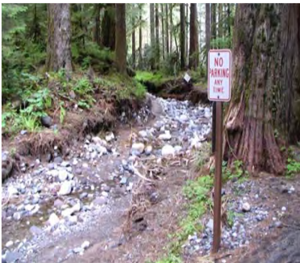
Photo 11: Ipsut Scour No Parking Any Time
