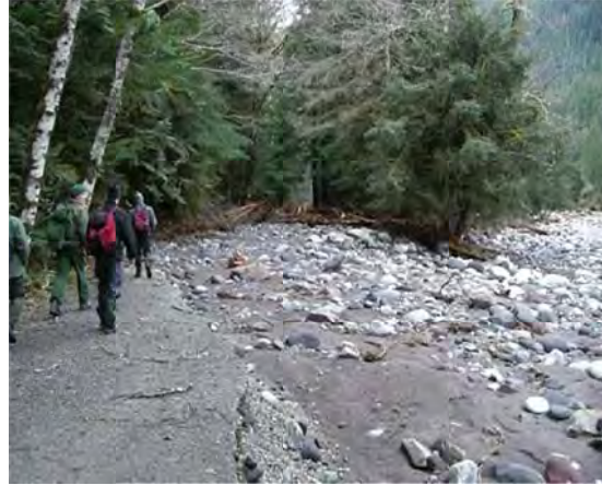
Photo 25: Section of Washed Out Road
