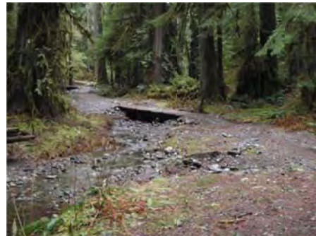
Photo 18: Scour Near Culvert on Carbon River Road
