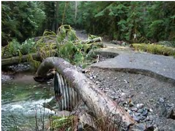
Photo 22: Ranger Creek Culvert
