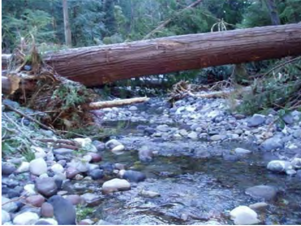
Photo 7: Falls Creek Washout
