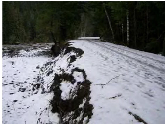
Photo 23: Sloughing Along Edge of Road
