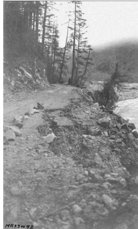
Photo 2: Early Slumping along the Carbon River Road
