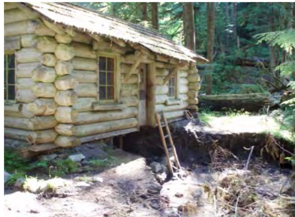
Photo 14: Ipsut Creek Patrol Cabin Undermined
