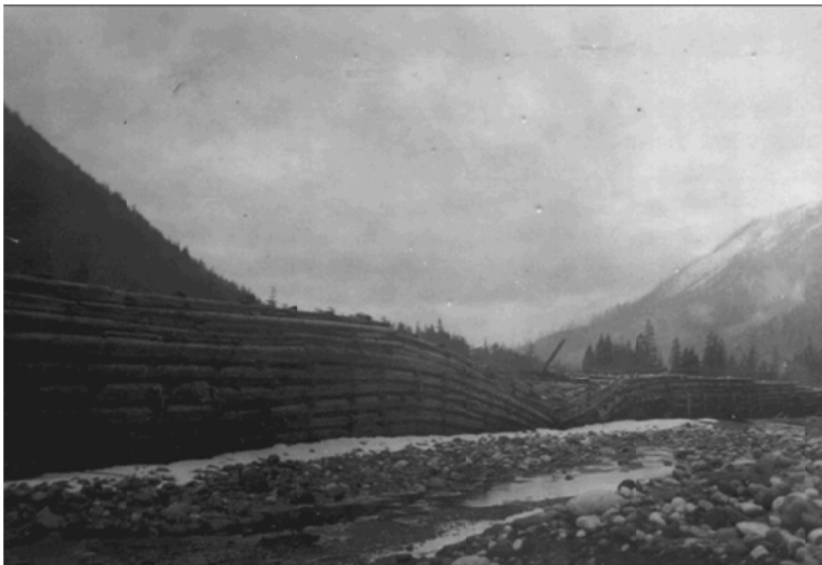
Photo 3: Carbon River Road 1930s Log-Cribbing
