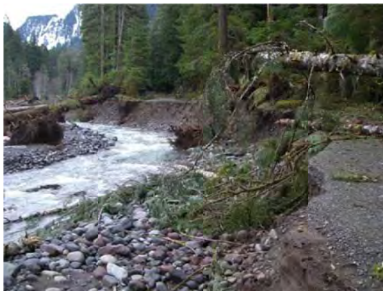
Photo 27: Milepost 4.4 (Looking Northeast)
