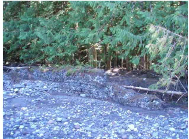
Photo 5: Cobble Gabions Near Falls Creek
