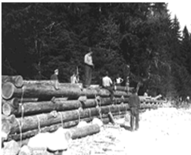
Photo 1: Log Cribbing Installed in 1930s along Carbon River Road
