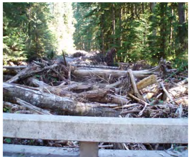
Photo 12: Ipsut Creek Bridge Logjam
