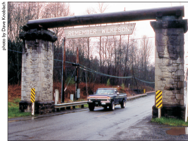
Figure K-3. The Wilkeson sandstone structure at Wilkeson before it was damaged by the 2001 Nisqually earthquake. The new structure was rebuilt in 2004 using the same sandstone blocks. View is to the north.
