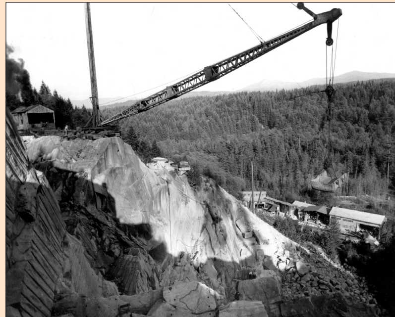
Walker-Wilkeson quarry in the late 1920s. A derrick that can move both equipment and rock rubble in the quarry lifts a container. The gang saws were in the shop buildings at the base of the slope. View is to the northeast. Photo courtesy of Tacoma Public Library.
