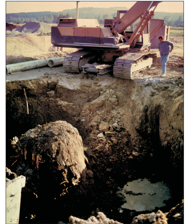
Figure J-5. One of the many large subfossil trees unearthed in 1993 during excavations for a sewer line at a new subdivision in Orting. This Douglas-fir was rooted about 16 ft (5 m) below the present land surface. Its average breast-height diameter was more than 9 ft (2.8 m). Tree-ring matching tells us that it was about 360 years old when it was buried by the Electron Mudflow from Mount Rainier at about A.D. 1500. The Electron began when a massive part of the upper west flank of Mount Rainier collapsed and began to flow as a wet, thick slurry at high velocities down the Puyallup River. While the average speed of the flow was about 30 mi (48 km) per hour, in the upper reaches of the river it flowed significantly faster. The lahar likely reached this area about one hour (or less) after it had been initiated at Mount Rainier. It was probably more than 100 ft (30 m) deep when it exited the Cascade Mountains near the present town of Electron, and likely flowed through the site of Orting as a surge about 30 ft (9 m) deep.
