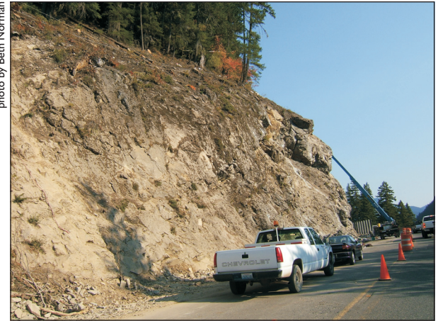
Figure H-6. Roadwork along an unstable slope where altered volcanic rocks adjacent to an intrusion (right) frequently collapse onto the highway. This outcrop is slightly east of MP 144 on the north side of the highway.
