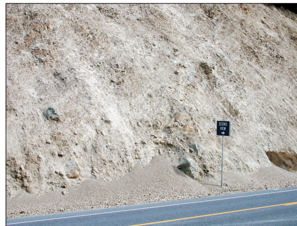
Figure H-10. Shattered rock of the pre-Tertiary Russell Ranch Formation is exposed near MP 148 along US 12. The Russell Ranch unit includes marine sedimentary and volcanic rocks that are at least in part of Late Jurassic and Early Cretaceous age (~145–130 Ma). The complex consists mainly of sandstones and mudstones with minor conglomerates, reworked water-lain tuffs derived from volcanic-arc volcanoes, and pillow lavas (altered to greenstones) that likely formed at an oceanic ridge (Miller, 1989).
