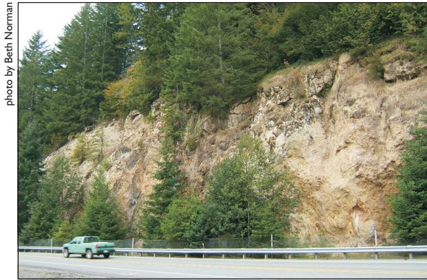
Figure D-7. Hydrothermally altered andesite along the north side of SR 410 slightly east of MP 38.
