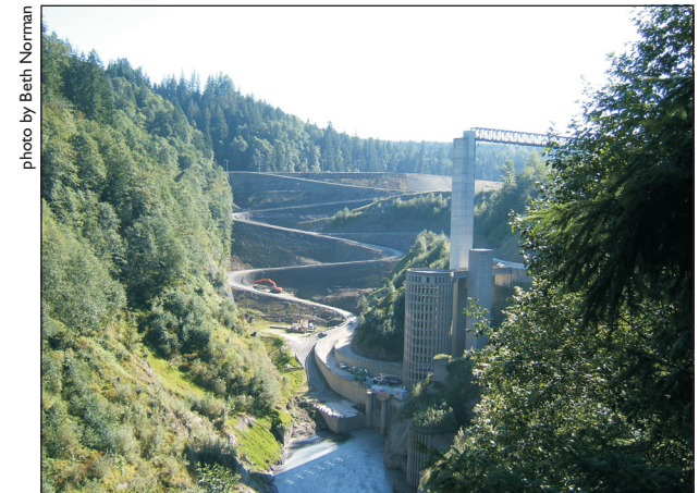
Figure D-5. Mud Mountain Dam. This earth-fill embankment dam was constructed for flood control in the lower White River basin.
