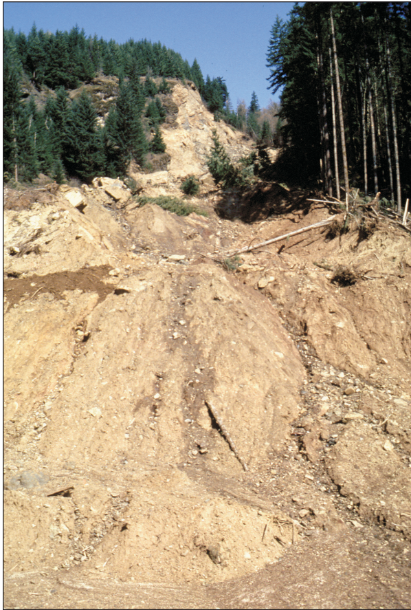
Figure C-13. A landslide complex north of US 12 about 1 mi (1.6 km) west of Randle at Peters Road. The failure occurred in stages at about 6:00 pm on Nov. 22, 1995. One landslide nearly hit a vehicle. This photo was taken in April 1996. During a period when the hillside was saturated, a zone of clayey gouge associated with a north-trending fault here failed when bedrock blocks from the cliff toppled onto upper slopes and overloaded the slippery material. The vertical distance from the topple to the road is about 800 ft (250 m). US 12 now goes around the toe of this slide.
