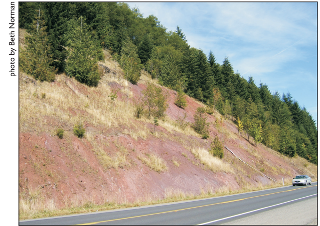
Figure C-4. Zone of reddish altered rocks. Slickensides are common on these sheared rocks, although no trace of a fault is visible.
