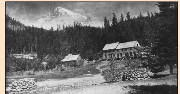
Longmire Springs Hotel, probably built 1906, with the southeast flank of Mount Rainier in the background and enclosed springs. Courtesy of University of Washington Libraries, Special Collections, photo 'nps longmire cabins'.
