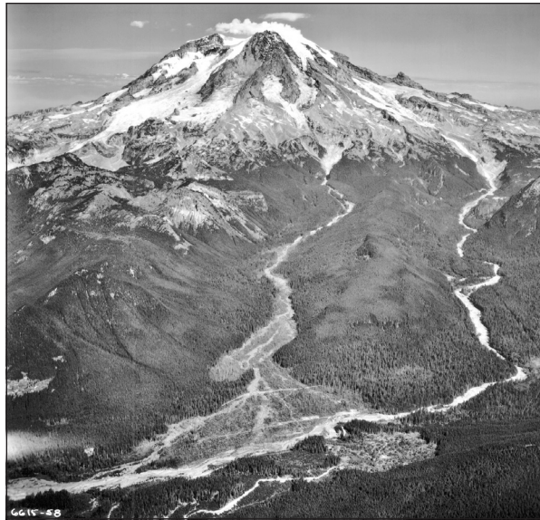
Figure A-16. Aerial oblique photo of Kautz Creek (center) showing the extent of the 1947 debris flow. This glacial outburst event temporarily dammed the Nisqually River (right) and buried the old park road under 20 ft (6 m) of rock and mud. In the flood of November 2006, Kautz Creek shifted its course about 0.5 (0.8 km) to the east. Photo by Austin Post, USGS, taken Sept. 22, 1966
